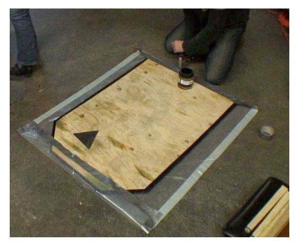
Staple it a lot! We used an excessive amount of staples and it worked well. Then duct tape over your staples, making sure to overlap over onto the plywood to seal it even better.
